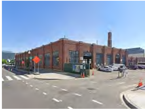
VIEW FROM FIRST ST & O ST
